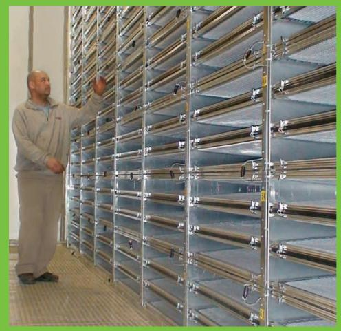
Above is a bank of Dynamic V8's in a 125,000 cfm custom air handler in a highrisk office application. These units are permanently mounted with front access.
