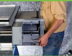
This is a slide out Dynamic V8 module in a filter box for a fan coil unit. These give a MERV 13 option for smaller equipment in LEED projects. This module was part of those that were installed throughout the LEED EB renovation of ASHRAE headquarters.
