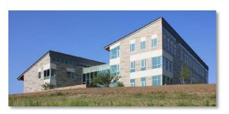
The majority of energy savings were in HVAC energy. These savings resulted from improved heating performance (heat pumps use ~25% of the energy that electric resistance requires for the same load), exhaust air energy recovery (reduces ventilation loads by ~70%), demand controlled ventilation (reduces ventilation loads by ~50%), improved envelope performance, and the decoupling of the outside air system from space loads which reduces reheat.
