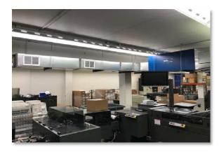
**Challenges:** Traditional filters used in the HVAC system serving the printing center were loading quickly with airborne particles generated by printing machinery and producing high system static pressures that necessitated expensive filter change-outs every two weeks. In addition to the high maintenance costs, the practices
